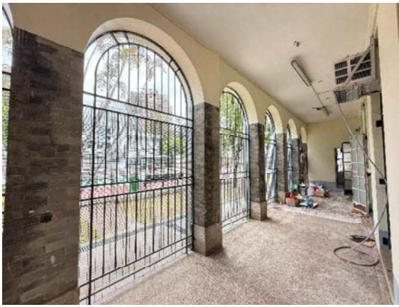
Fig 2.7.4 The open colonnade and arched verandah on G/F.
