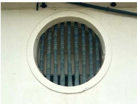
Fig 2.7.14 The circular porthole window.
