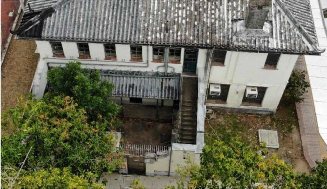
Fig 2.6.2 Aerial photo of Block P (North-East).
