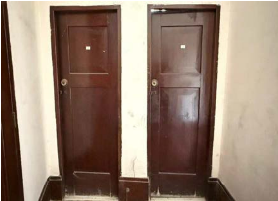
Fig 2.8.12 The original toilet cubicle doors.
