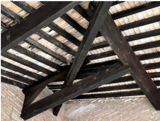
Fig 2.7.8 Trusses and purlins as roof structure.
