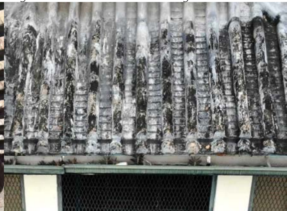
Fig 2.7.9 The roof tiles laid in a double-roll-double-pan style.
