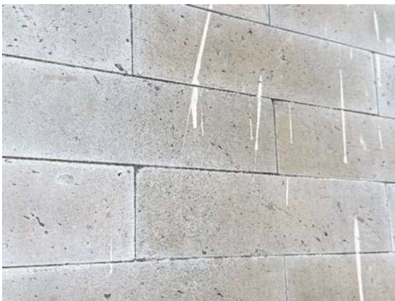
Fig 2.7.21 Jointless grey gauged brickwork at Block P Kowloon Hospital
