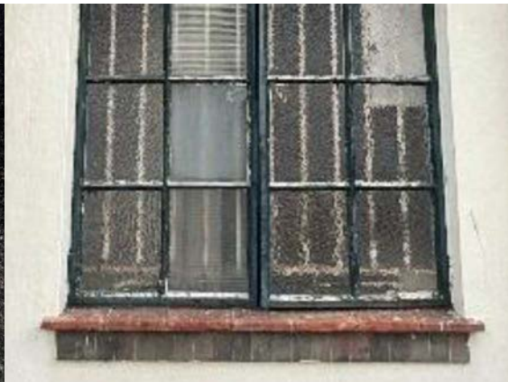
Fig 2.7.11 Jointless grey gauged brick window trims.
