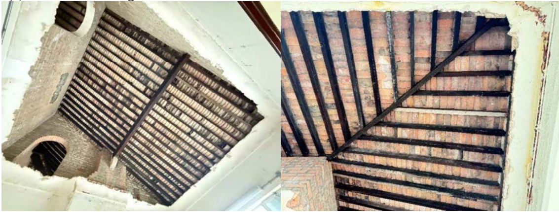
Fig 2.8.22 & 23 The original timber ceiling has been removed, leaving the roof exposed.
