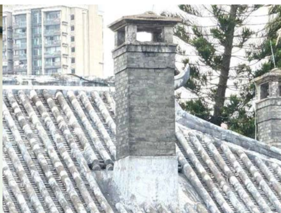
Fig 2.7.15 The chimney stack.
