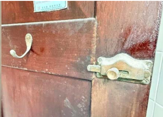
Fig 2.8.13 The ironmongeries at the door.
