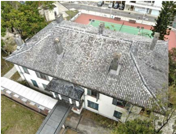
Fig 2.7.6 The Chinese tiled hip-and-gable roof.
